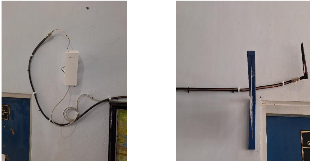
Figure 4. Leaky Feeder Implementation
